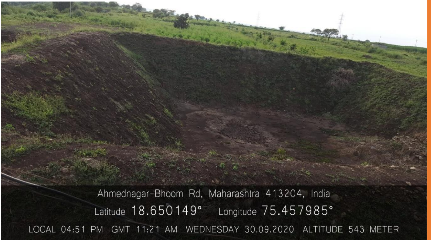
Farm Pond build at Planed college
